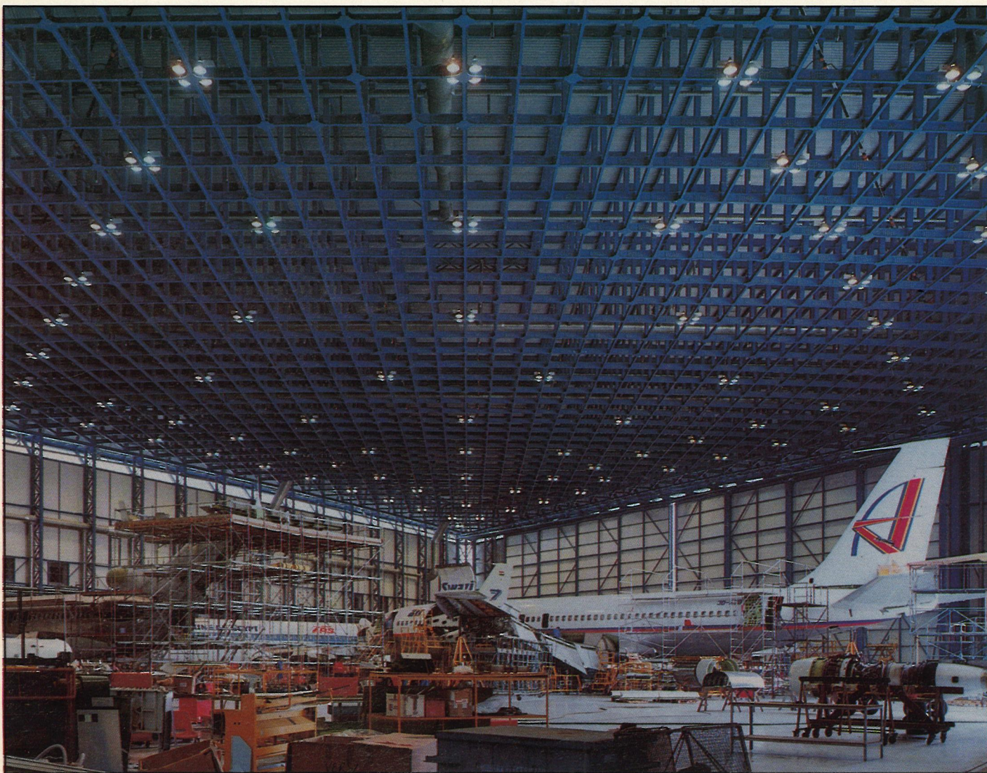
Stansted Airport — Simplex high bay fittings, using SON and MSI lamps, provide good but cost-effective lighting with good colour rendering.
