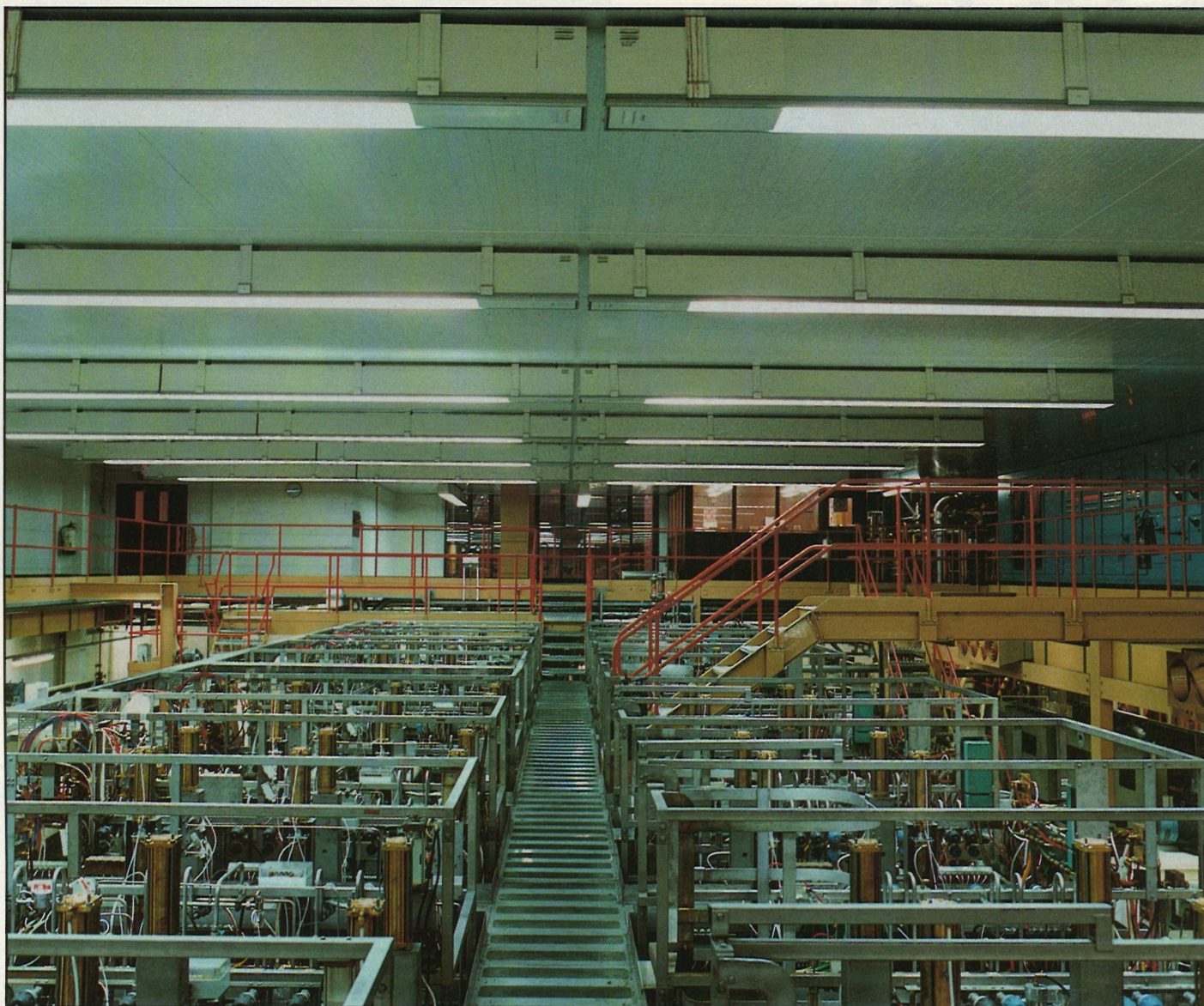
Bass brewery — Conductalite luminaires mounted back to back allow access to lamp and gear units from a single point. Each pair of luminaires provides glare-free illumination over the process area.
